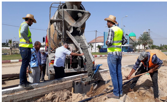
Casting concrete foundations for electrical poles in northern side of GIE
