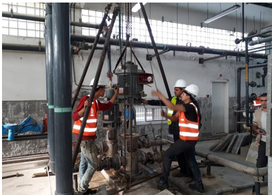
Dismantling the high-pressure pumps for the desalination
