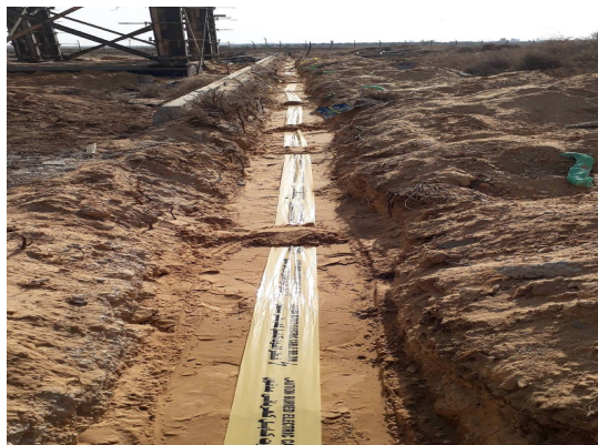
Installing underground 3" PVC flexible for poles in northern side of GIE
