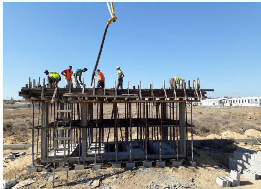
Casting ribbed slab for transformer room
