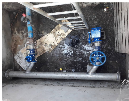
Installation of new manifold for sewage substation works
