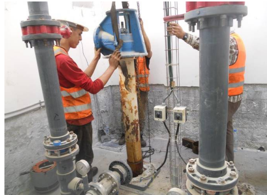
Dismantling the existing High-Pressure pump for maintenance
