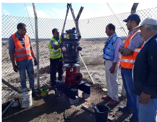
Installation of Vertical Turbine Pump for water well
