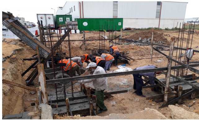
Casting of foundation of transformer room
