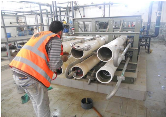
Dismantling the existing RO membranes
